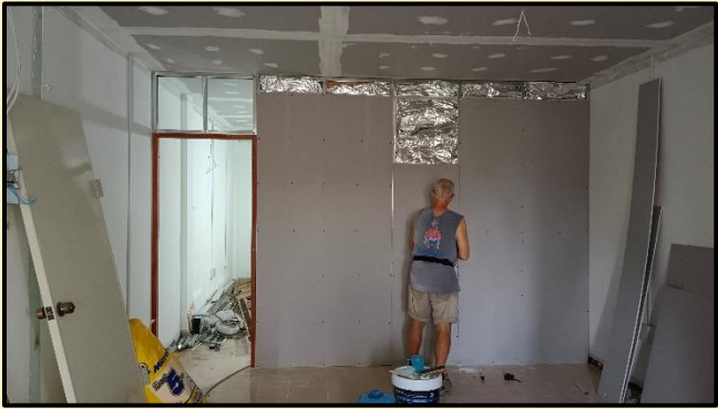
Mike volunteered to put up the wall on the 3 rd floor.
