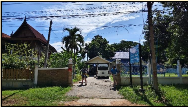
The main electric wire sparked when it rained.
