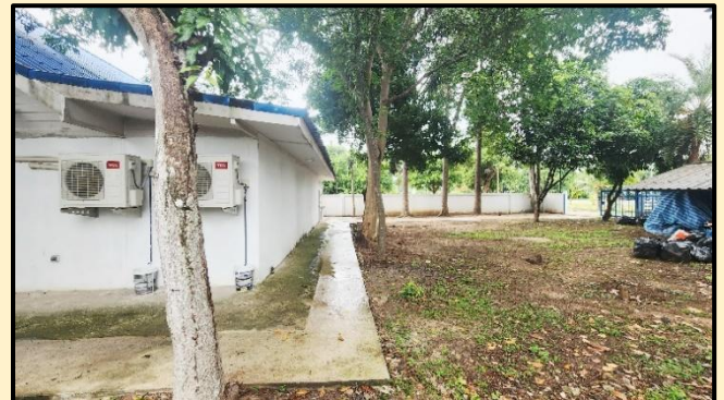
We need to add covering for this walkway.
