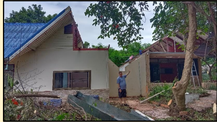
We need to repair the roof and build a meeting room.
