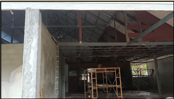
The new roof gives more space for 2nd-floor rooms.
