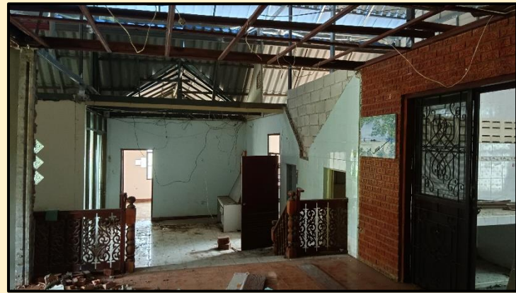
The 1 st floor rooms need ceilings and paint.
