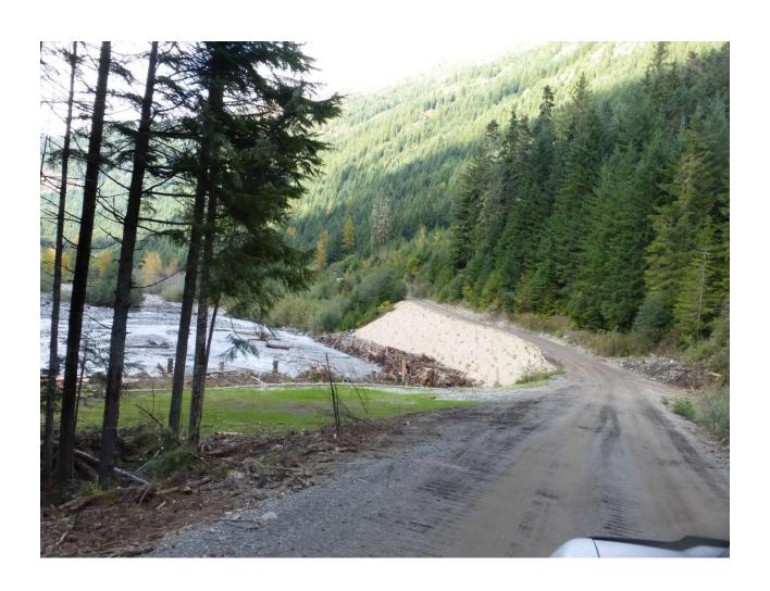
East Church FSR 3040 MP 1.0, 2015 Channel Flush out Power House Company Cleaning up site to standard. Prevented road erosion from misdirected water flow.
