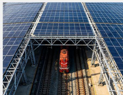
Photovoltaic panels above railway tracks
