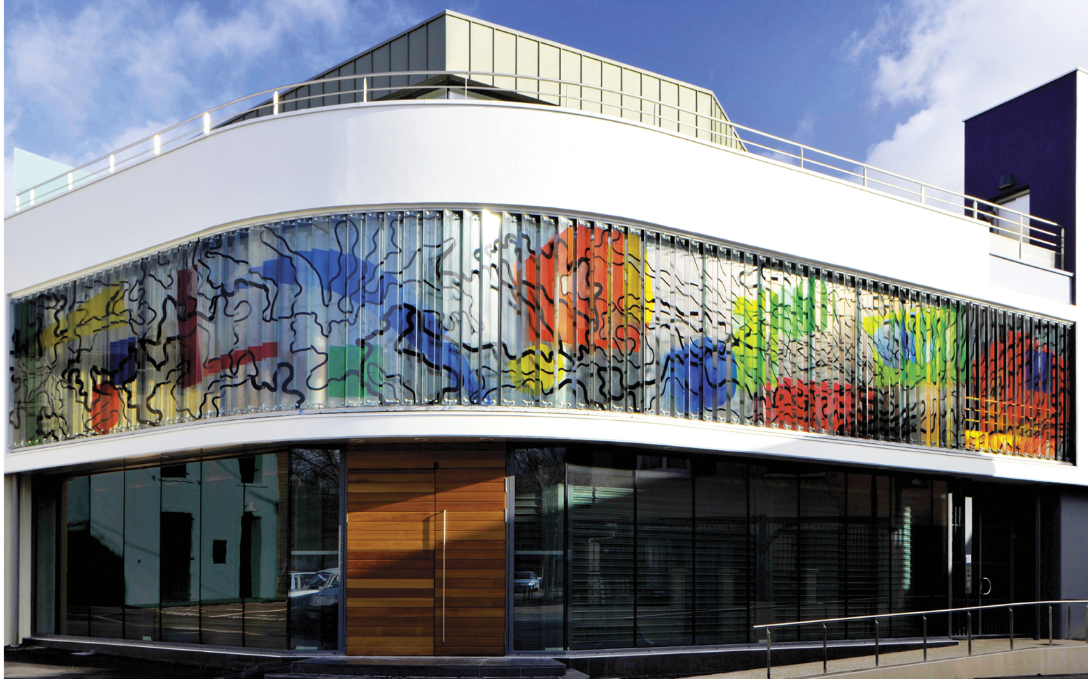
Architecte: Vial Gaivoronschi
