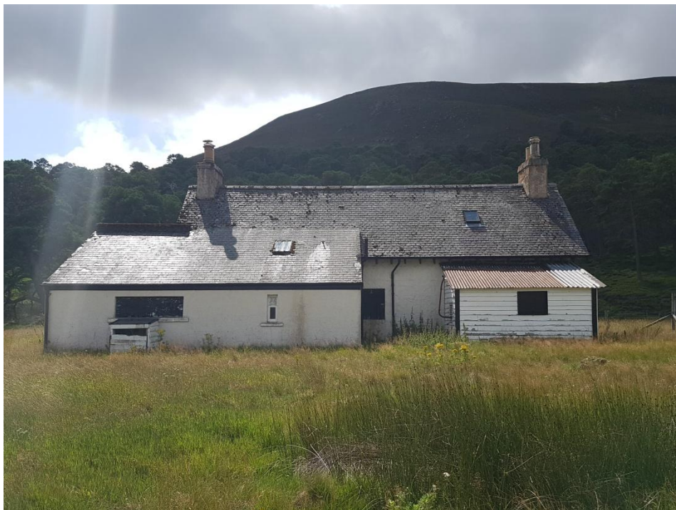
Old Keeper's Cottage
