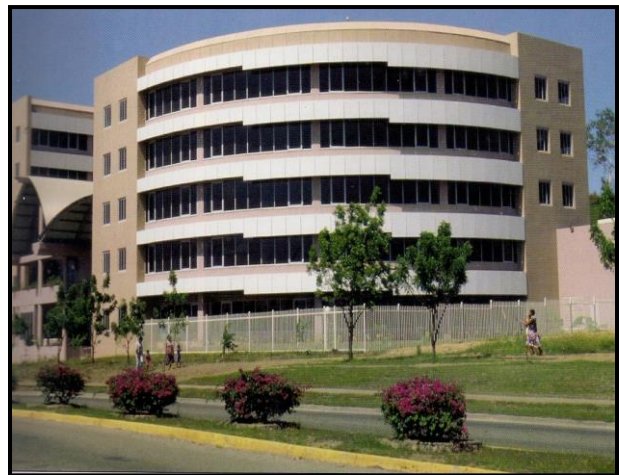
Five story building in Waigani, Port Moresby
