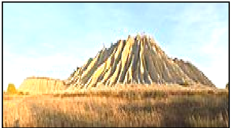
A spoil tip covered in rills and gullies due to erosion processes caused by rainfall
