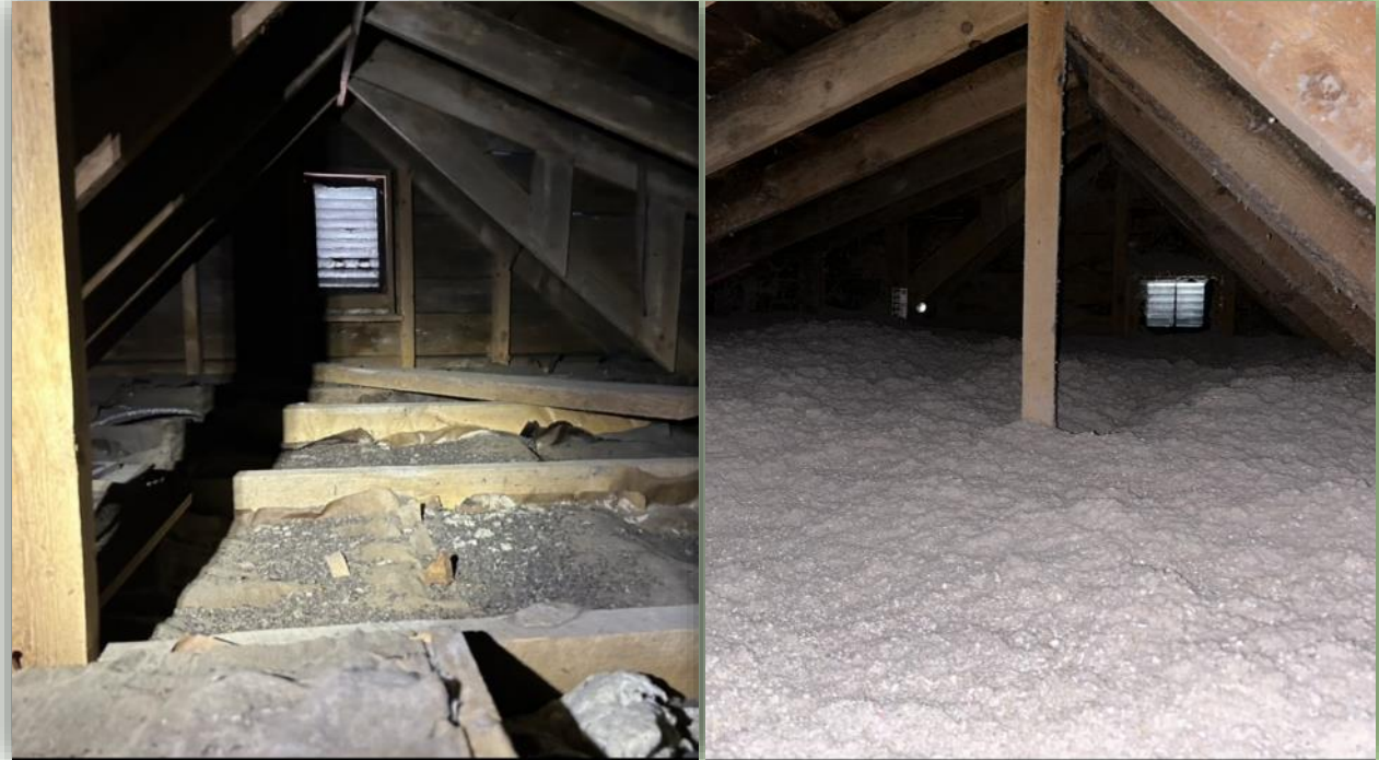
Attic before and after air sealing & insulation
