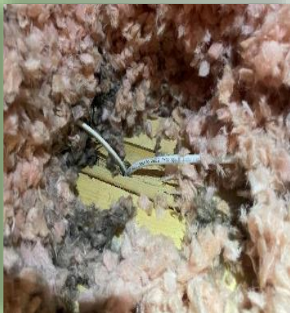
Pipe & electrical penetrations
