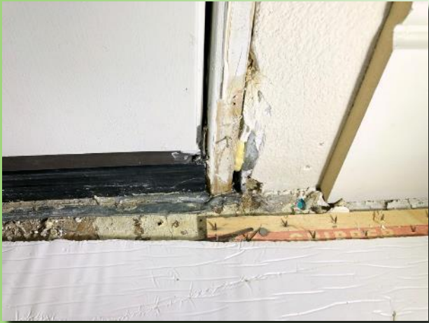
Cracks around exterior doors
