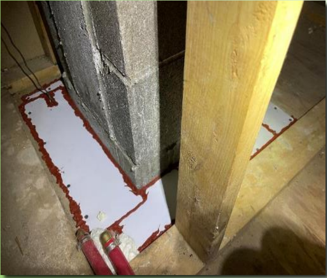
Air sealed chimney chase w- fire-rated materials
