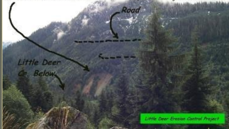
Example of a Slide Caused by a Deteriorating Road
