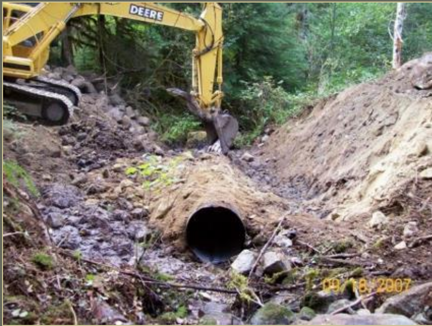
Undersized Culvert
