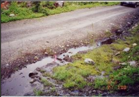
7/20/00 Rd 36 Mile 3.24 Installed culvert
