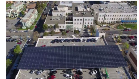
Kaiser Permanente Richmond Microgrid
