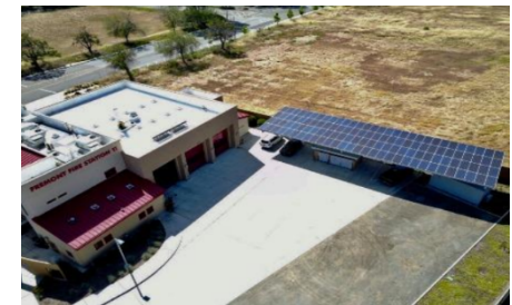
Fremont Fire Station Microgrid
