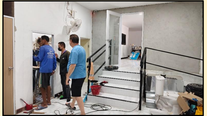
We renovated the bathroom and the worship room wall.
