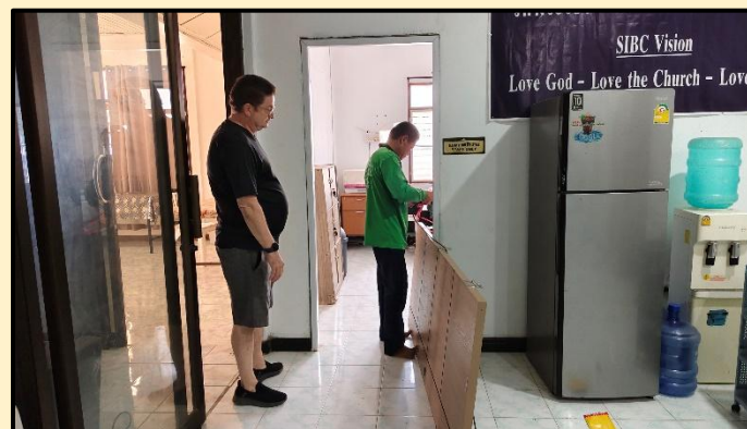
We replaced 3 doors for the office and 2 classrooms.
