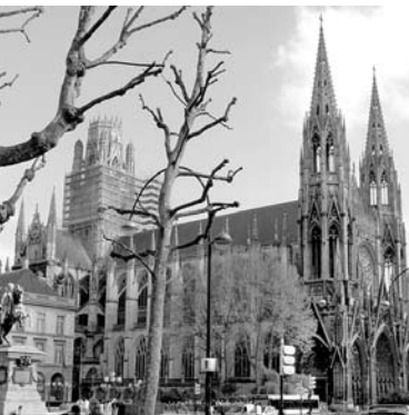
Exterior of Saint-Ouen
