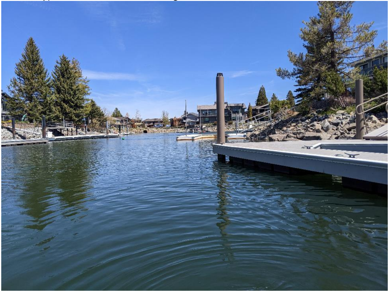
Photo 4. Typical conditions in the West Lagoon – Site 1
