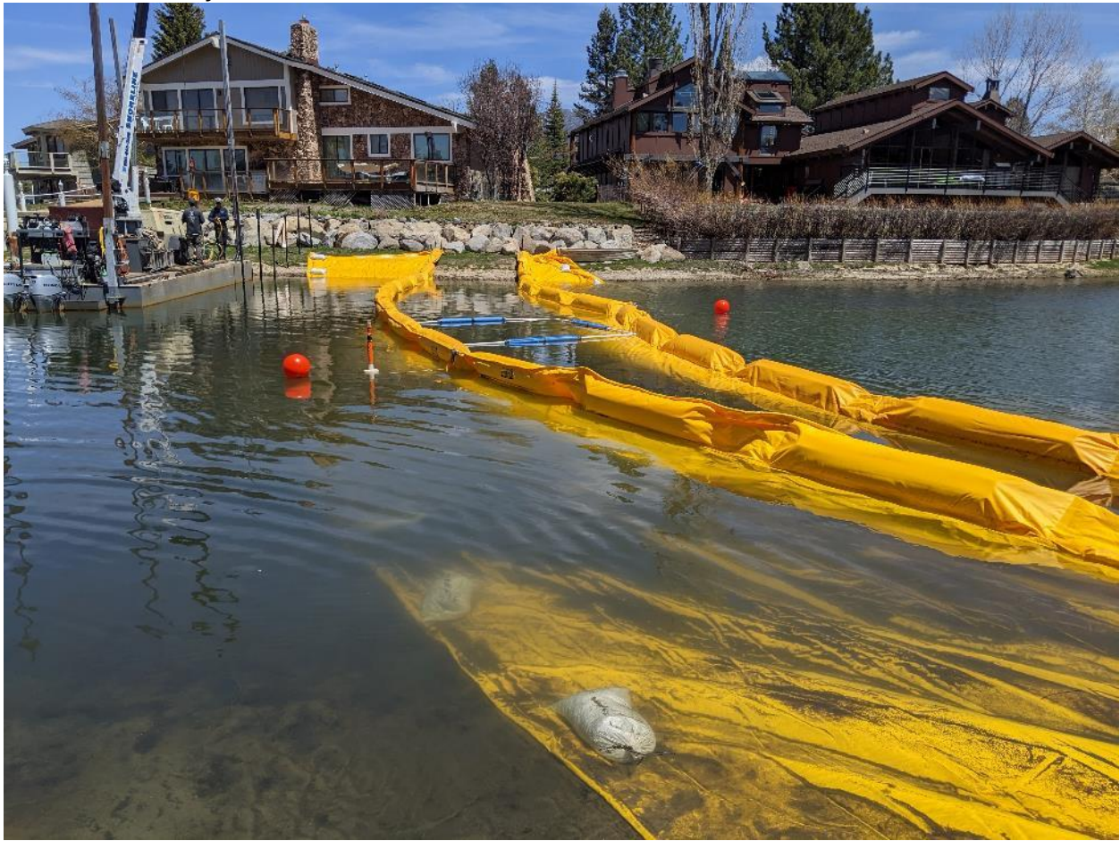
Photo 7. Turbidity curtain installation north of Site 15
