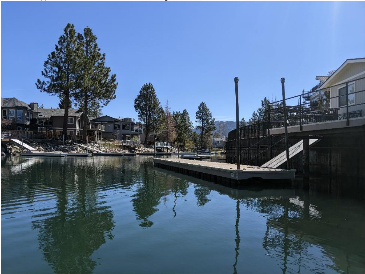
Photo 1. Typical Conditions in the West Lagoon with seawalls and rocked banks
