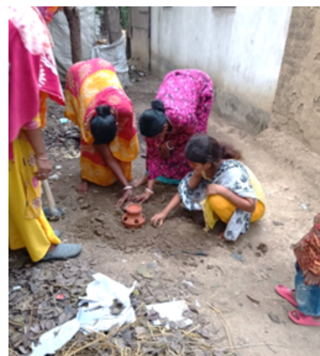
Matka installation for eco-friendly sanitary disposal at Paschim Medinipur
