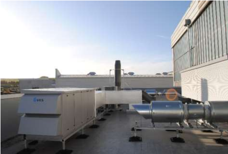
Example AHU Installation
