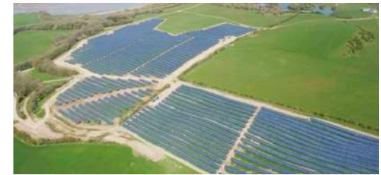
ROANHEAD, UK 7 MWp
