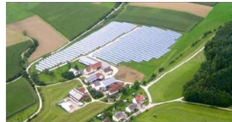
WOLPERSTETTE, GERMANY 2.2 MWp
