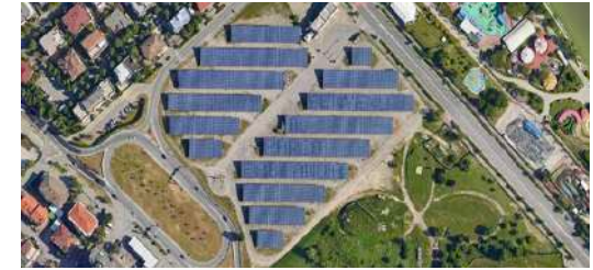
REMINI, ITALY 1.8 MWp
