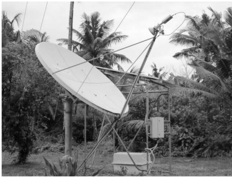
This is an actual Vsat that was installed by Telikom PNG in Aua village, Manus Province.
