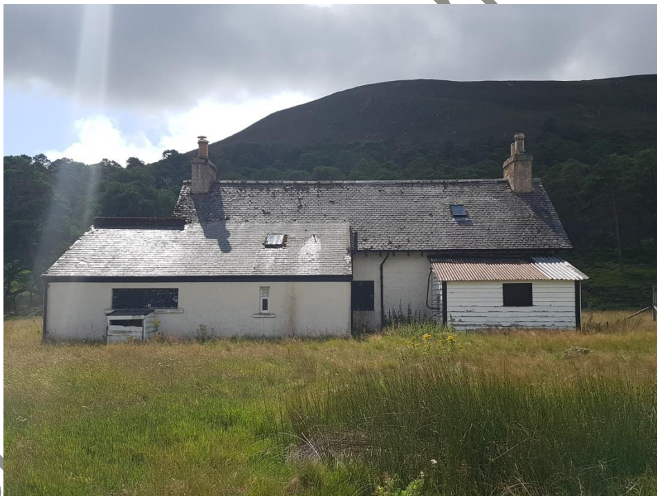
Old Keeper's Cottage
