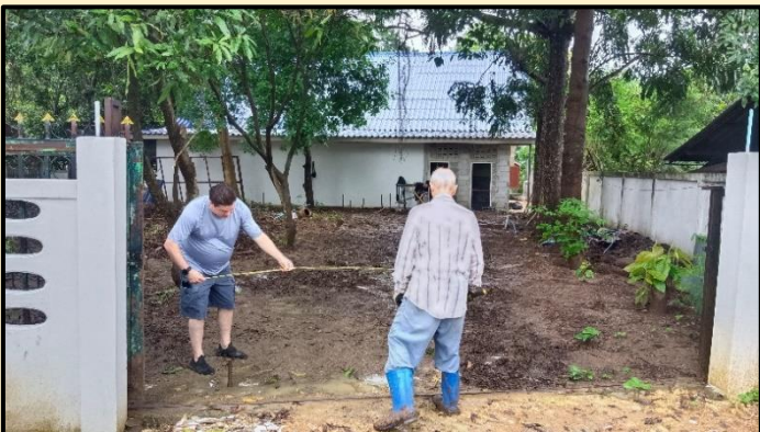
We will make the cement path to the worship room.
