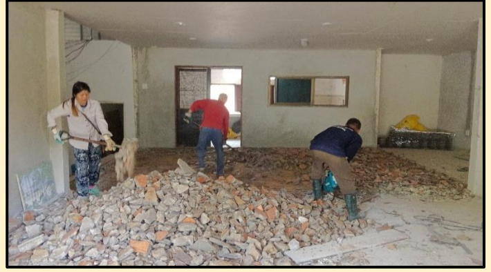
A couple and a friend broke the tiles and removed them.
