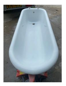
We then paint on an epoxy primmer which we allow to cure for between 24-48 hours creating a solid bond with the bath. We then sand this down in preparation for three coats of polyurethane high gloss top coats. Each coat is aloud to cure for 24 hours.
