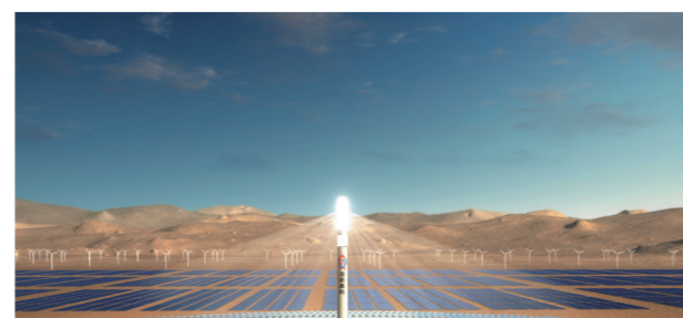
Jiuquan Suzhou 100MW Energy Storage Project S-3450/37kV Oil-immersed Transformer
