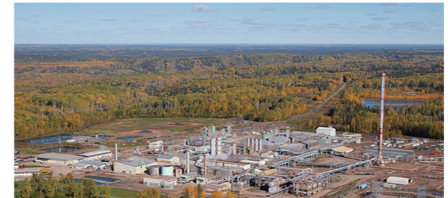
Canada 1000m³ Hydrogen Project ZHSZCB-5800/35kV Hydrogen Production Dry Type Rectifier Transformer
