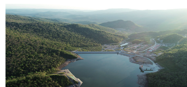
Changjiu new materials Pumped-storage Project KSG-1000/10kV Mining Dry Type Transformer
