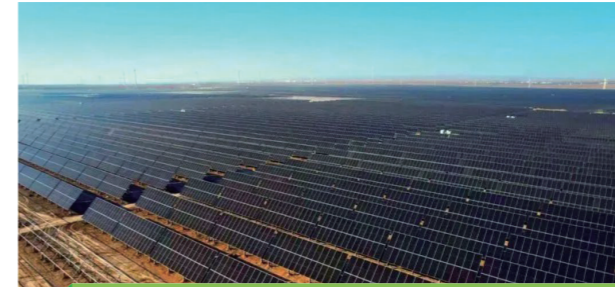
Gansu Minqin 42MW/84MWh PV Energy Storage Project SC(B)-2500/35kV Cast Resin Dry Type Transformer
