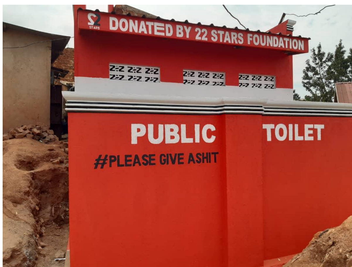
8 we build this toilet block opposite of our office in Kampala.
