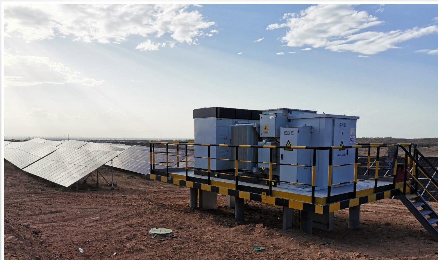
1500V 3.125MW Outdoor Inverter Solution
