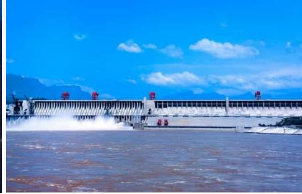
The Three Gorges Hydroelectric-Complex Project
