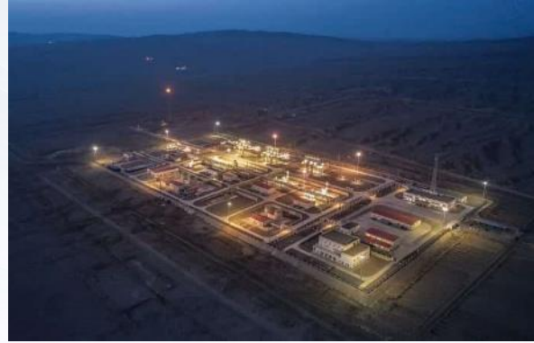
West-East Gas Pipeline Project
