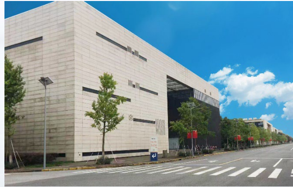
2023 Information Park B15b Data Center Optimization and Transformation Power Supply Project of Shanghai Telecom
