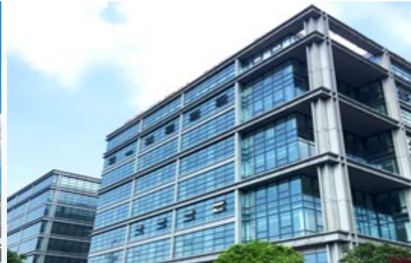
BAIDU Changzhou Data Center
