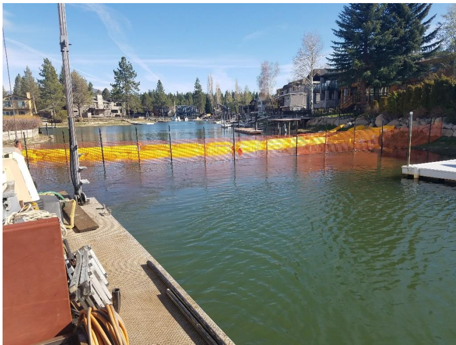
Turbidity curtain in Tahoe Keys as part of the control methods test has now been removed with herbicide levels at non-detect status.
