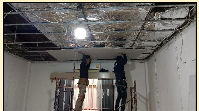
The workers are installing a new ceiling.
