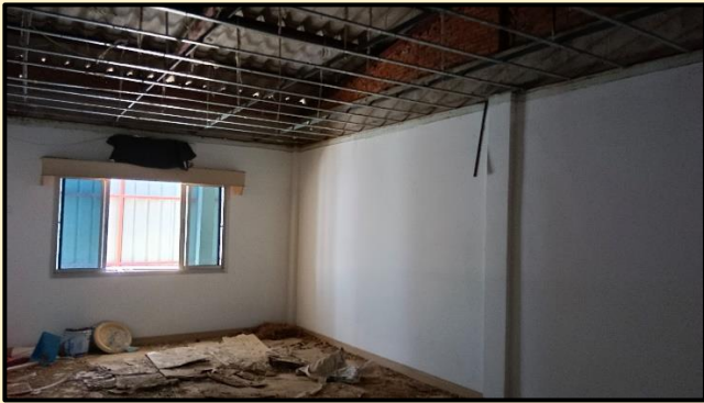
The 3 rd floor ceiling of both sides were pulled down.
