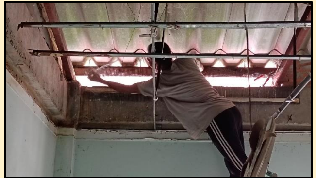
Putting screen to stop pigeons from living in the attic.
