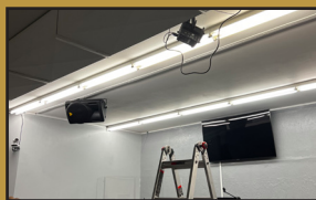
New lighting installed
