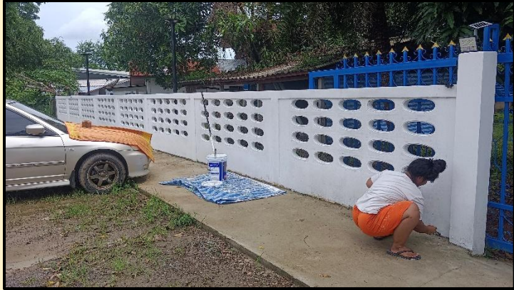
We painted the front wall at the parking lot.
