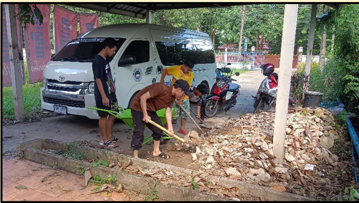
These bricks were moved to fill in veranda foundation.
