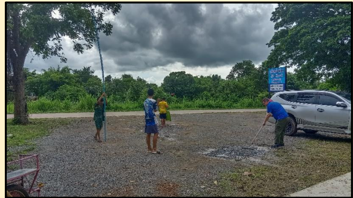
More gravel was put on the parking lot.
