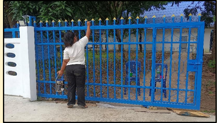
Both gates were painted to make them look new.
