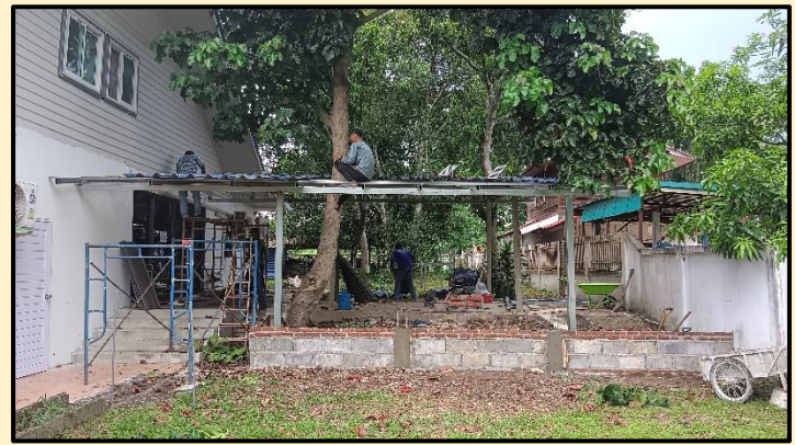
We extended its foundation and roof.
