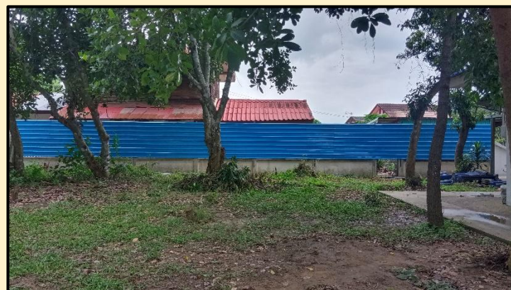
This wall was set up for more privacy.
