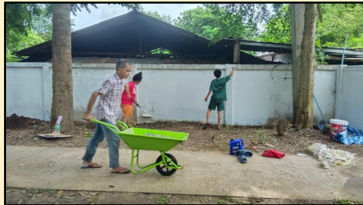
The walkway wall was painted. The gravel was taken out.
