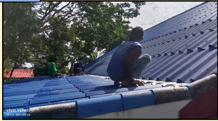
All the leaks on the roof were filled up.
