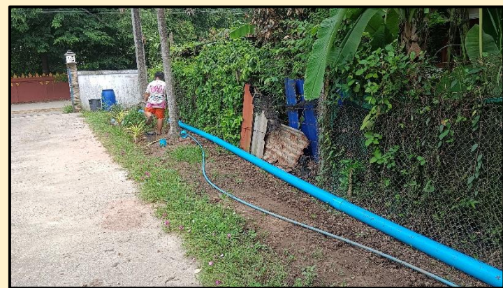
Joy connected the big drain pipes to the city's drain.
