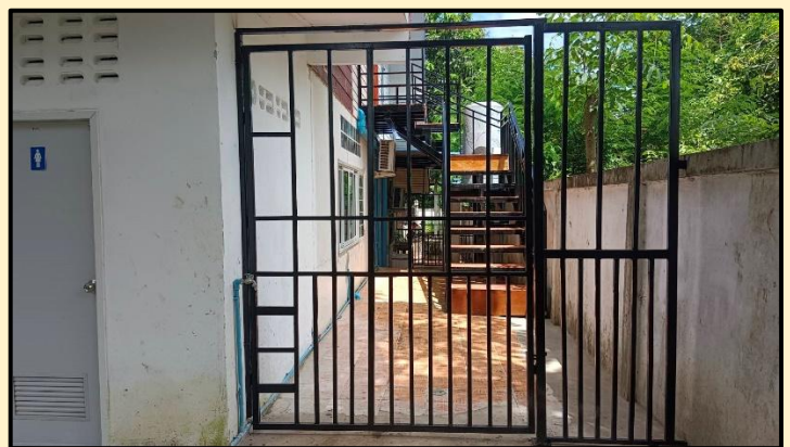
The gates of both sides will secure the upstairs area.
