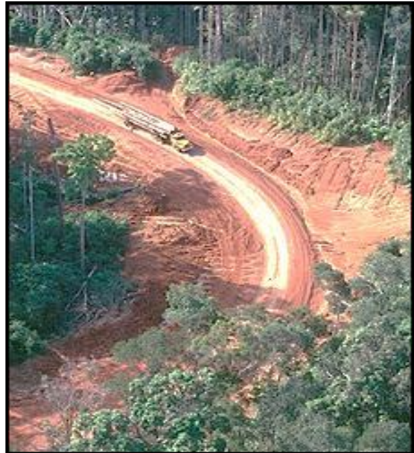
A Newly Cut Road for transporting timber
