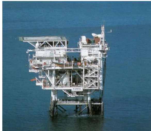
Kumul terminal in Gulf – this is where crude oil is loaded onto tankers to be transported to refinery sites.
