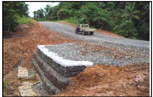
Kiunga - Kokonda Road after construction, North Fly District, Western Province.
