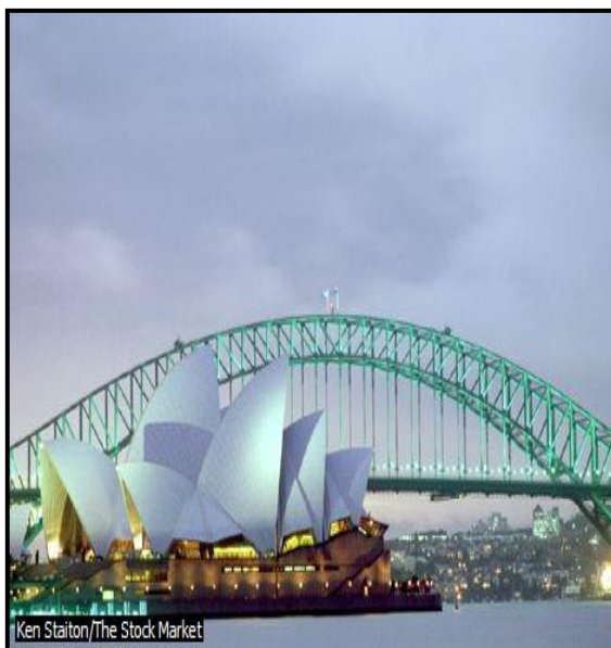
Sydney harbor Bridge
