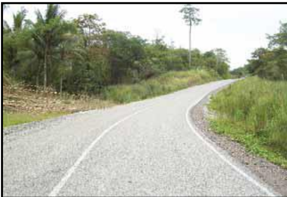
Completed section of road, Ormond Bridge to Bukuku along Magi Highway, Central Province.
