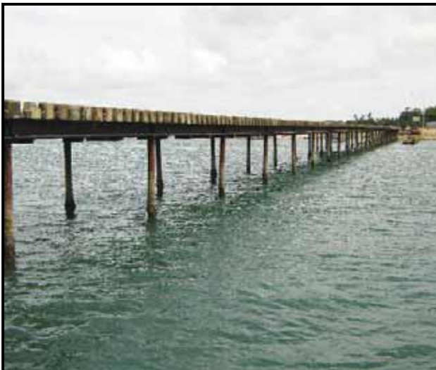
Daru Trestle Wharf, South Fly District, Western Province.
