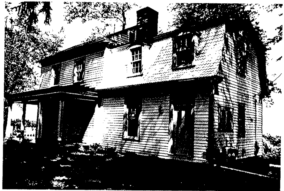
Conway Grove after Restoration.
