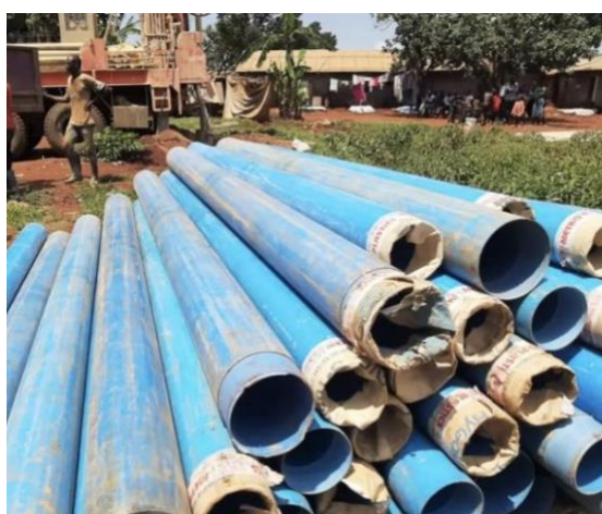
18. This was when the drilling started.
