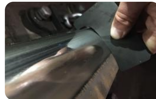
Rail side wear
