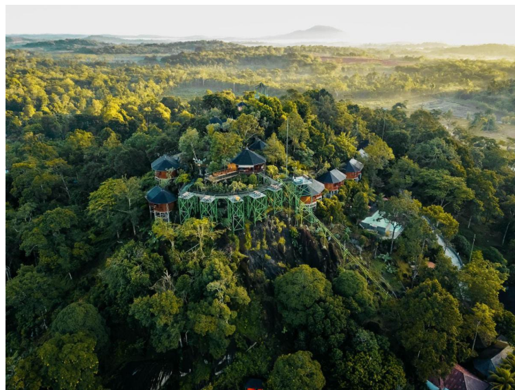
Utilise the site's natural setting to form a unique backdrop to future development; where possible, explore carbon potential
