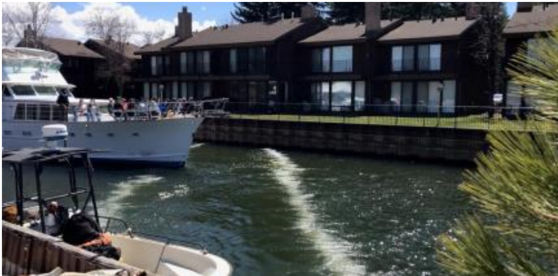
Figure 7. East Channel Double Bubble Curtain
