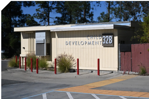
Outdated classrooms Grossmont College, Child Development Center
