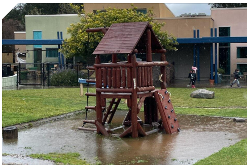
Drainage and flooding issues Cuyamaca College, Child Development Center
