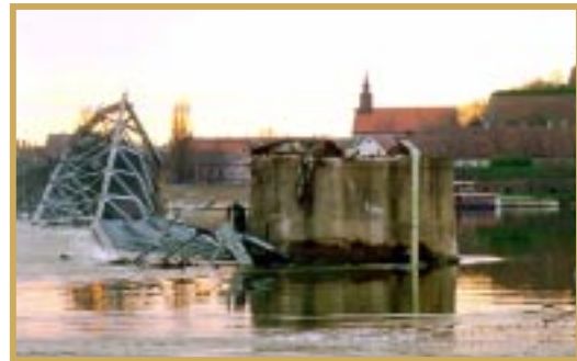
WATER SUPPLY LINE in Novi Sad, Yugoslavia, was destroyed along with this Danube River bridge during a NATO airstrike in April 1999.
