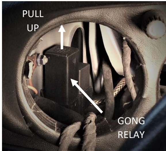
Figure 2 Gong Relay is behind fuel gauge
