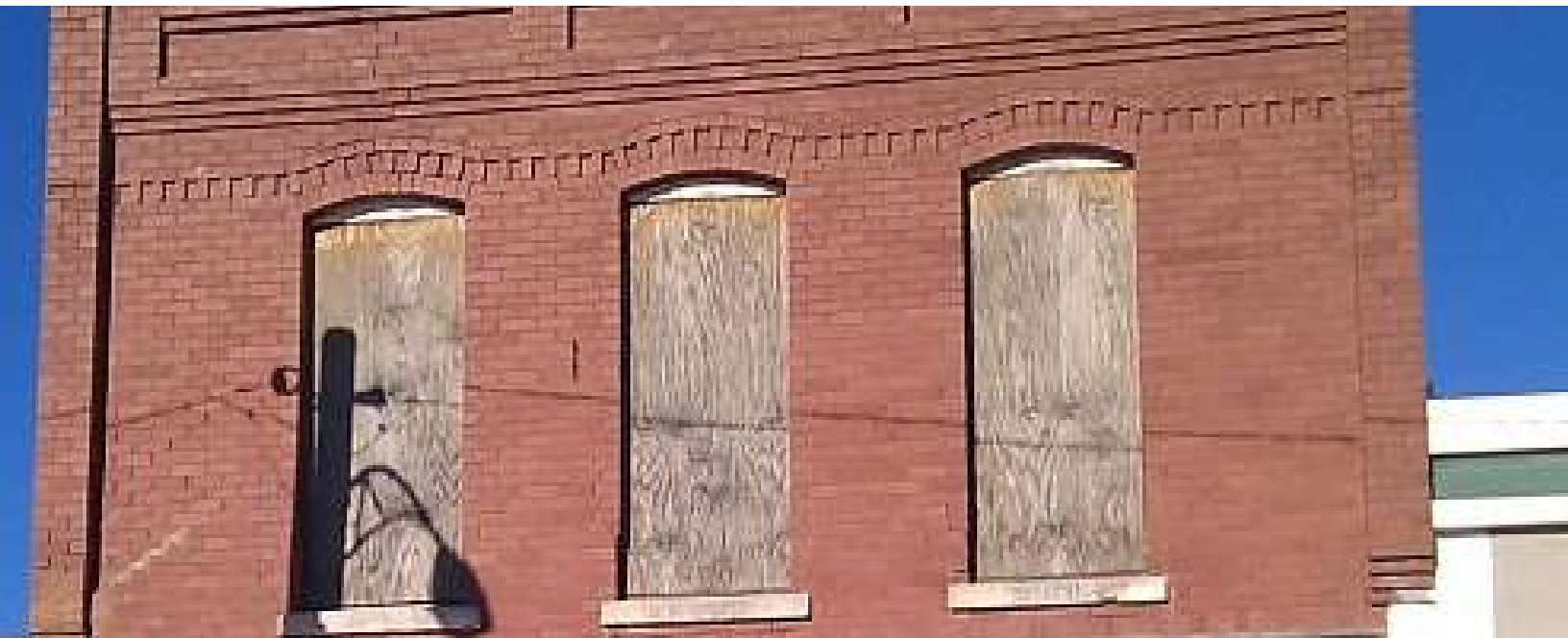
Vacant Building, Photo Courtesy of: City of Warren
