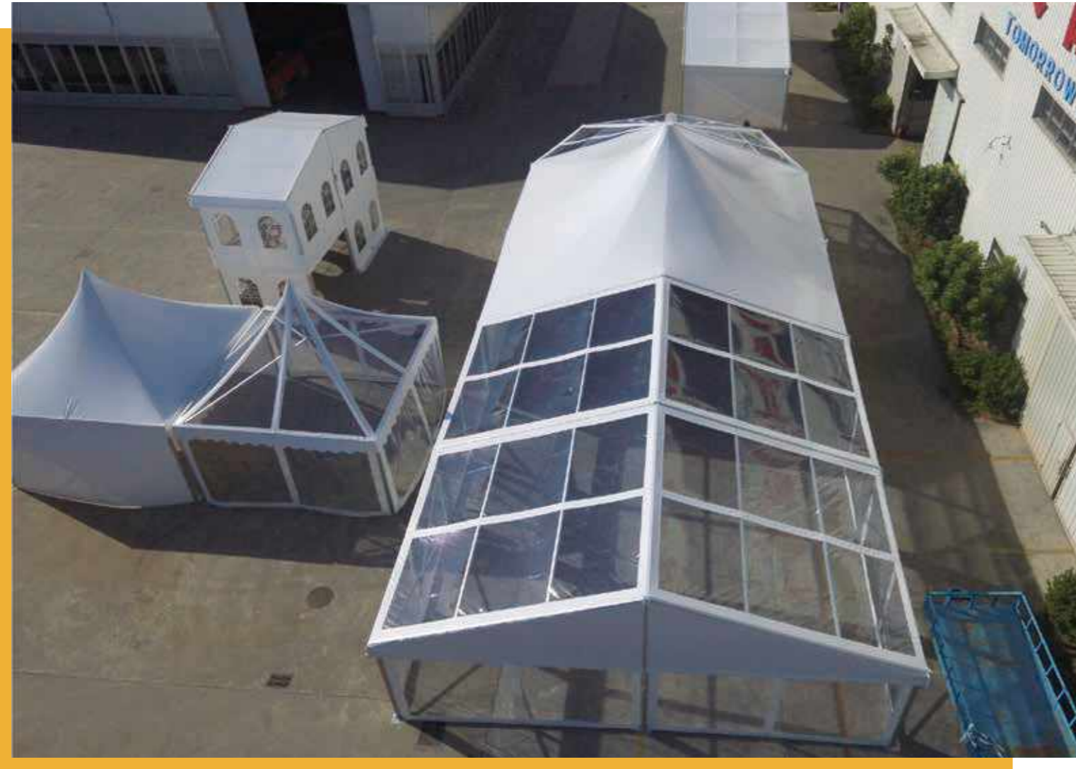
篷房顶布 Tent roof fabric(850g/m 2 , 0.6mm thickness)
